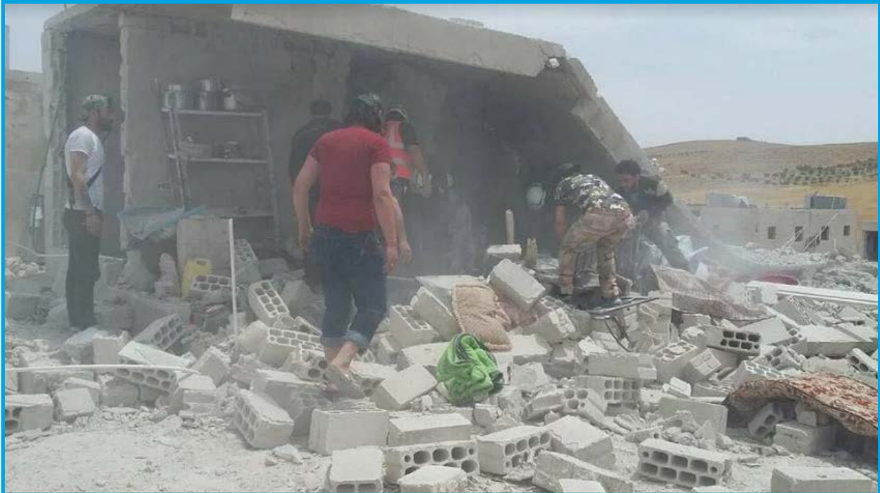
Destruction in the residences of al Shayyah area after the airstrikes by Syrian regime forces – April 30, 2017
