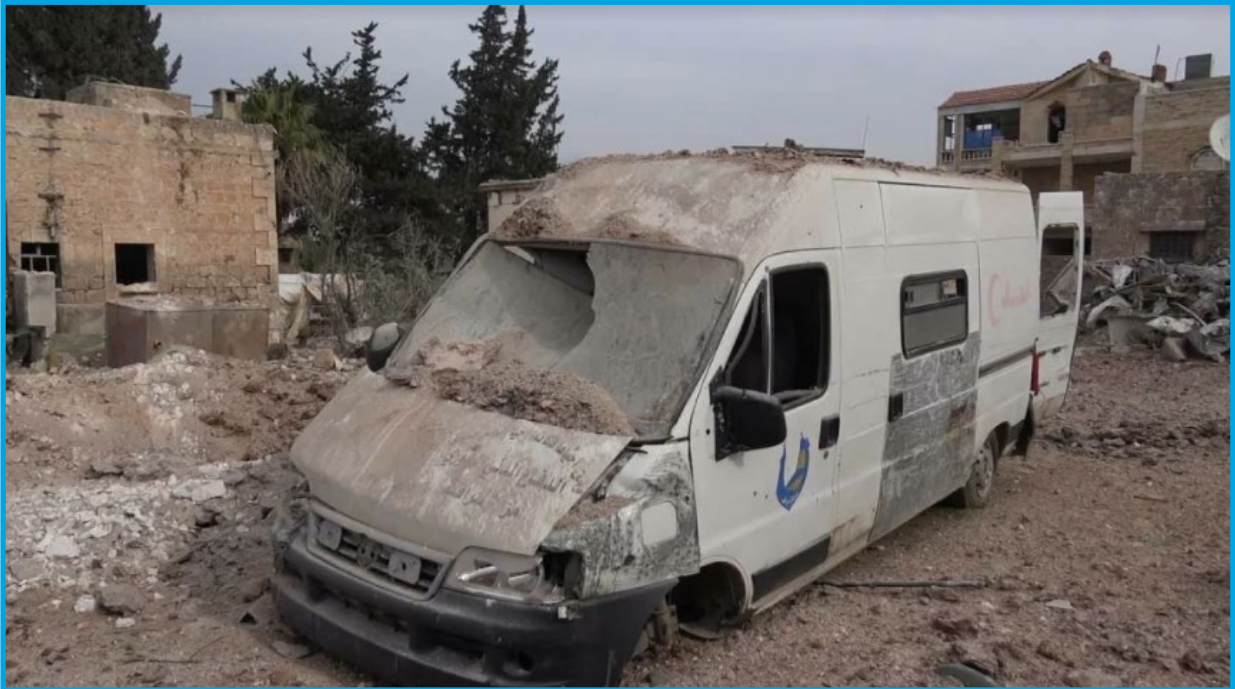
Damages to an ambulance in the aftermath of a bombing by warplanes we believe were Russian on the civil defense center in the middle of Sarageb city, Idlib – January 20, 2018
