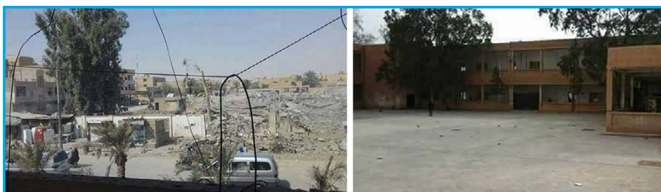
A picture showing Faye Mansour School in al Bokamal city, Deir Ez-Zour before and after it was bombed by international coalition forces – August 11, 2017
