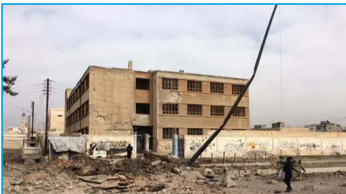
The destruction in Qurtoba School in al Wa'er neighborhood, February 26, 2017
